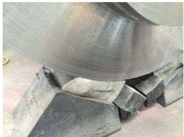
The rubber pads were scarce for the narrow flange. But there are no vibrations were transferred to the space.
