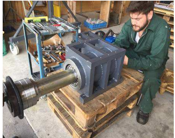
Picture 55: No hammer during installation, all with mounting auxiliary devices
