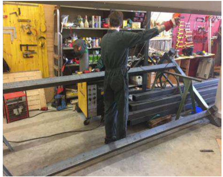
Picture 31: Frame welding
