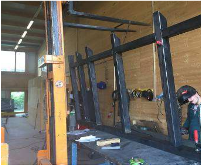
Picture 73: Jim during welding of the parts shelf subframe
